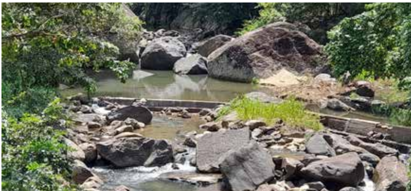
Construction of an anicut (small dam) at Watekgama to meet the water requirements of farmers in Owathanna and Kubagathanna paddy fields.
